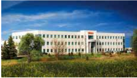
Mitutoyo America Corporation Corporate Headquarters Aurora, Illinois USA
